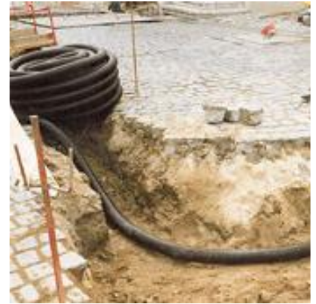
Kabuflex R and Kabuflex R-UV – provide advantages in inaccessible terrain and on uneven ground
