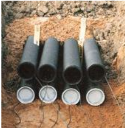
Kabuflex S – spacers indicating the direction make installations fast and safe
